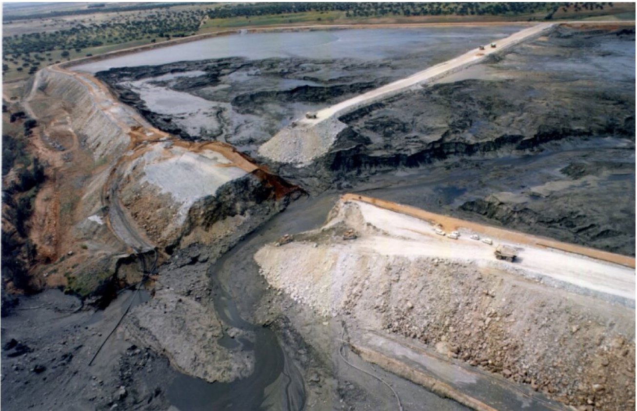
Fig. 6 Breach produced by the failure
